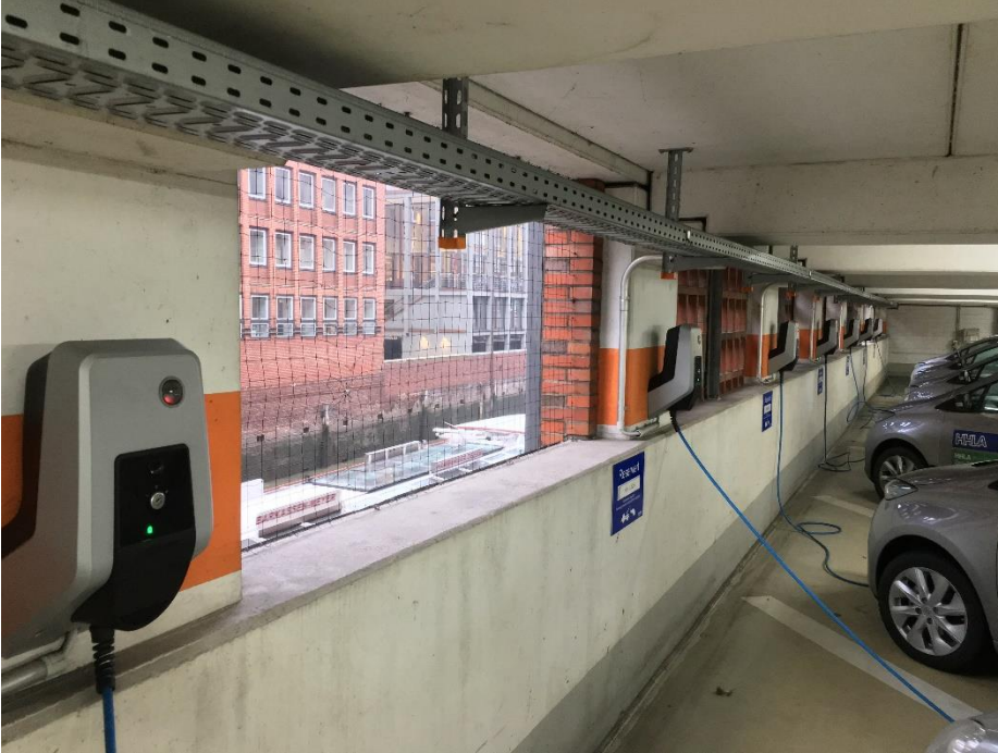
Parking garage Hamburg warehouse district
